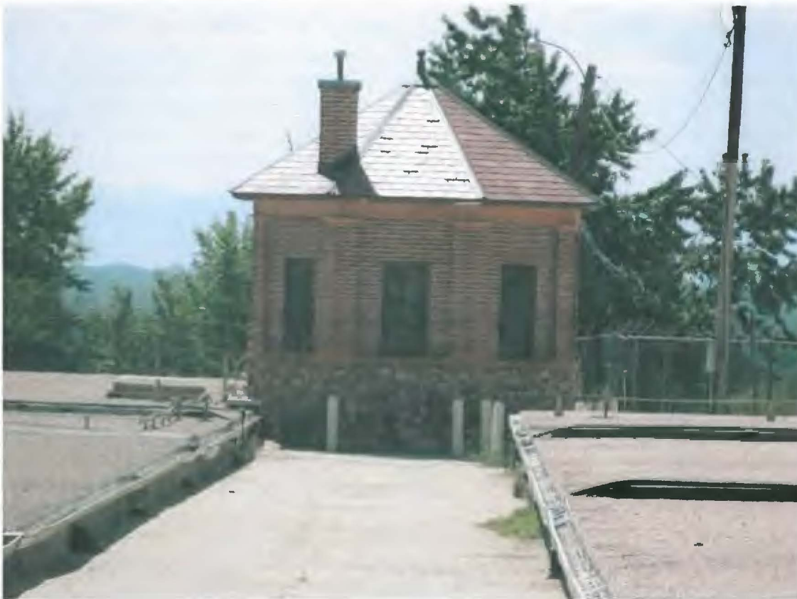
View of well- house from W. 30 th Avenue
